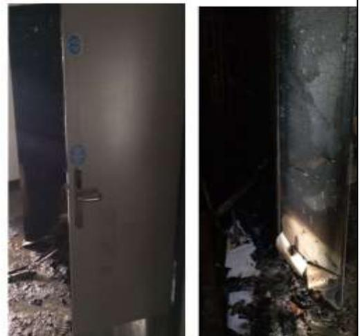
the paint has not blistered. The inner face of the door is heavily fire damaged but still intact.
