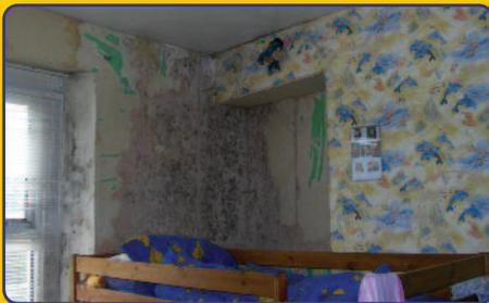
Severe condensation in this bedroom has caused the wallpaper to fall off the wall. Opening the window a little and heating the room adequately should help reduce the problems in this room.
